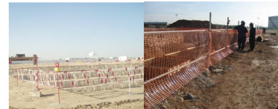
Barricading Excavation Areas
